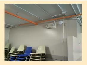
**Sprinklers** are in the process of being installed at Town Hall. In the lower level and some offices, the exposed pipes, which arrive in orange color, will be painted to blend in. In the Main Hall and addition, the pipes will be installed out of sight in the attic,
